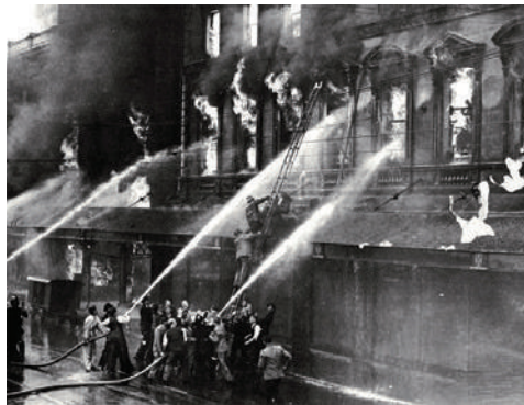
Ballantynes fire, Christchurch, 18 November 1947. Alexander Turnbull Library
