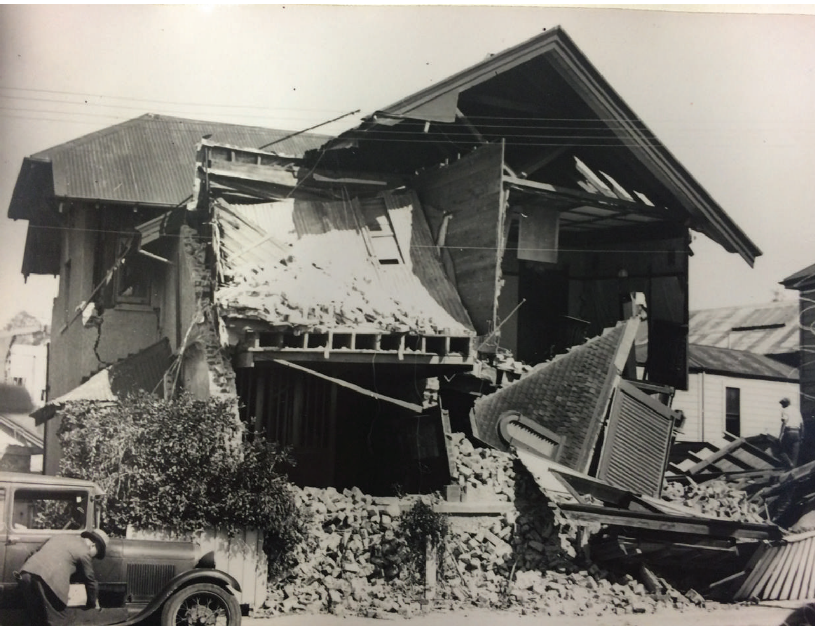
Napier earthquake, 1931. Alexander Turnbull Library.
