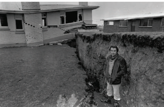
Abbotsford Landslide, 1979. www.teara.govt.nz
